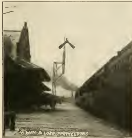
GRAVIT'S TRAIN ORDER SIGNAL "PROCEED" BOTH DIRECTIONS.
